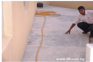
Figure 5: The Roof Surface
